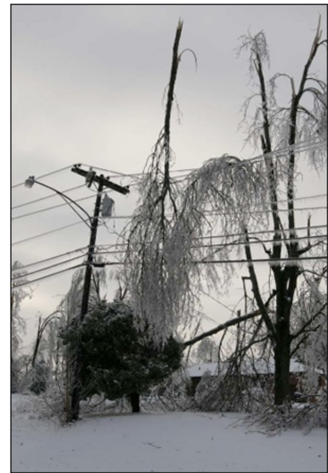
2009 Ice Storm Damage. Photo courtesy NWS Paducah website
