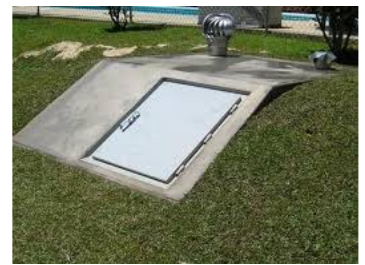
Left: Schematic home tornado shelter. Right: Surface view of a home tornado shelter in Dallas, TX.
