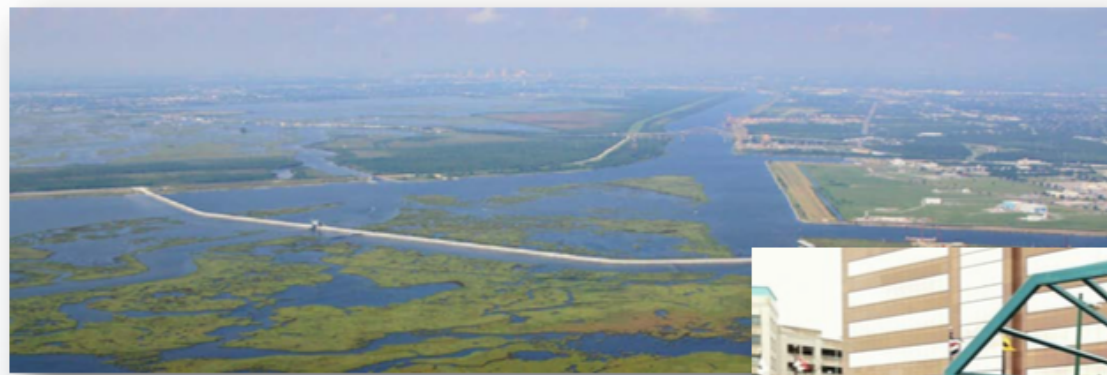
Storm Surge Barrier New Orleans
