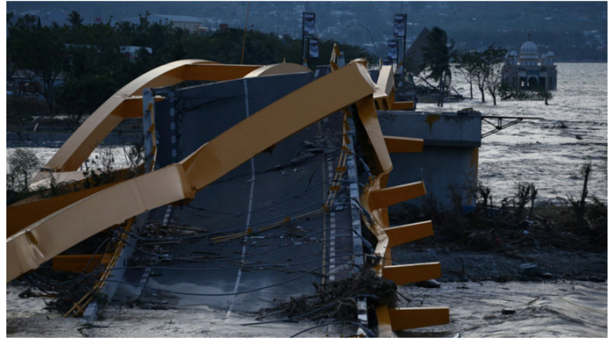
A bridge was wrecked at the city of Palu, after an earthquake and tsunami hit the area in Central Sulawesi, Indonesia. Athit Perawongmetha/Reuters
