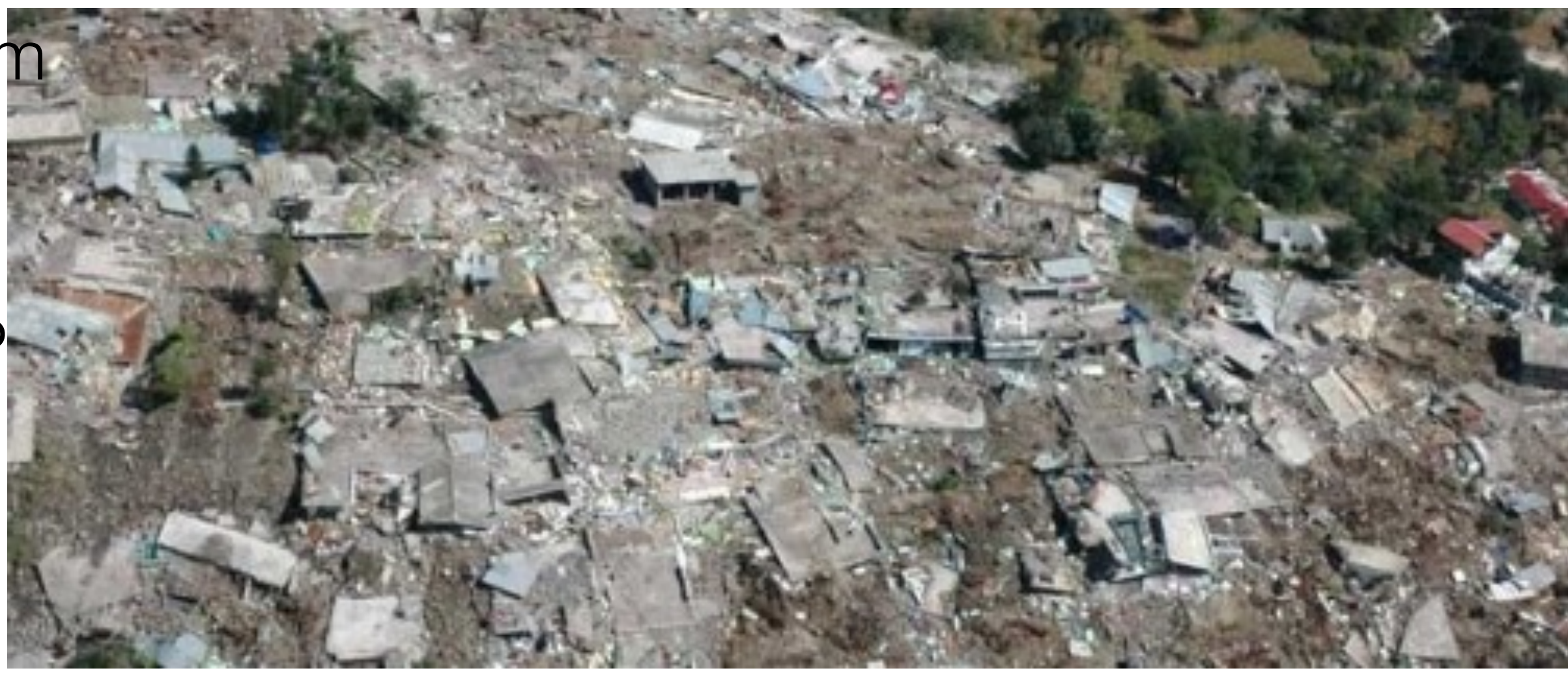
Destruction in Punjab, Pakistan Kashmir, caused by 23 seconds of ground shaking during the October 2005, Mw7.6 earthquake.
