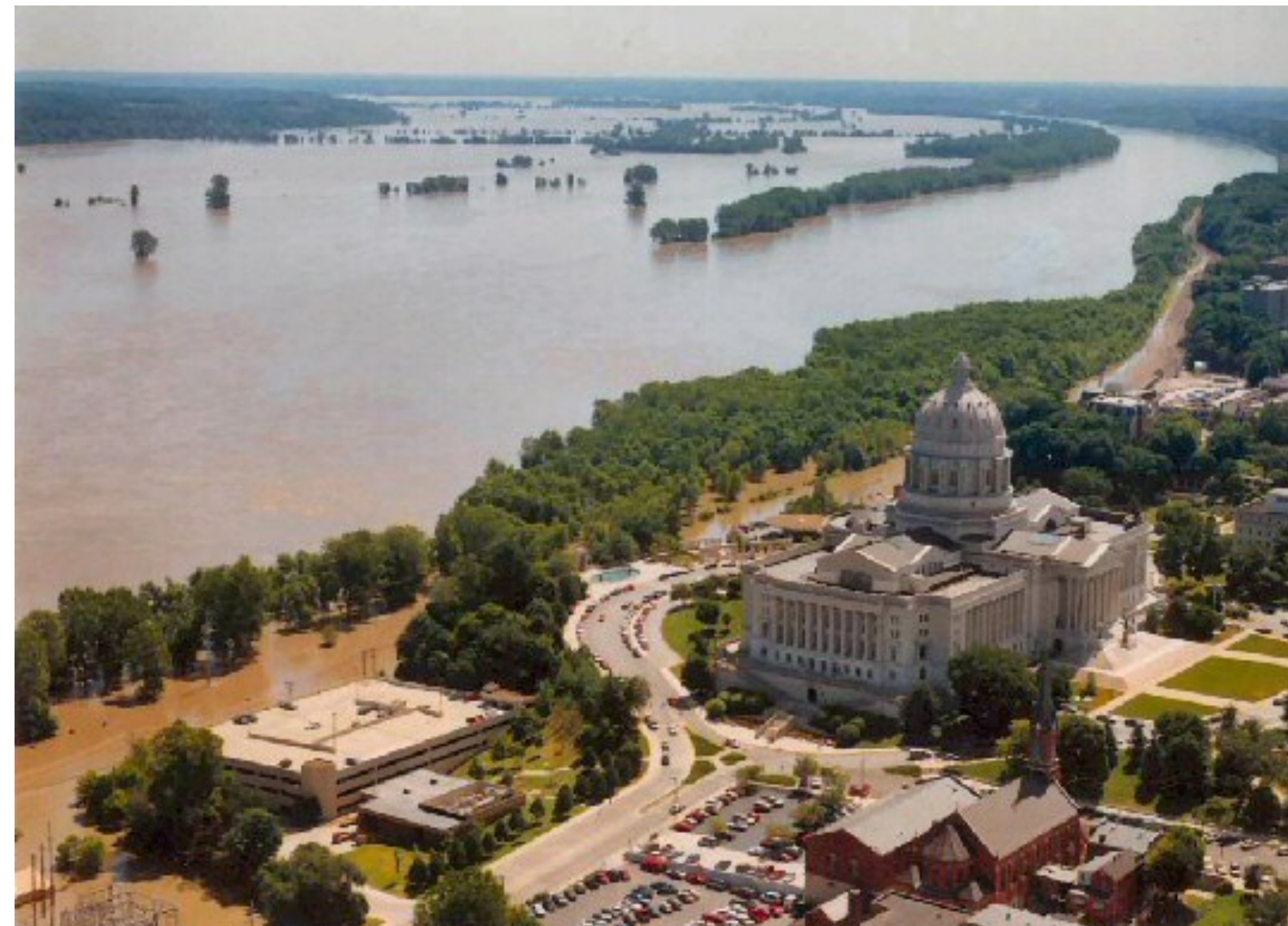
Jefferson City, Missouri, near the Missouri Capitol building during the "Great Flood of 1993".
