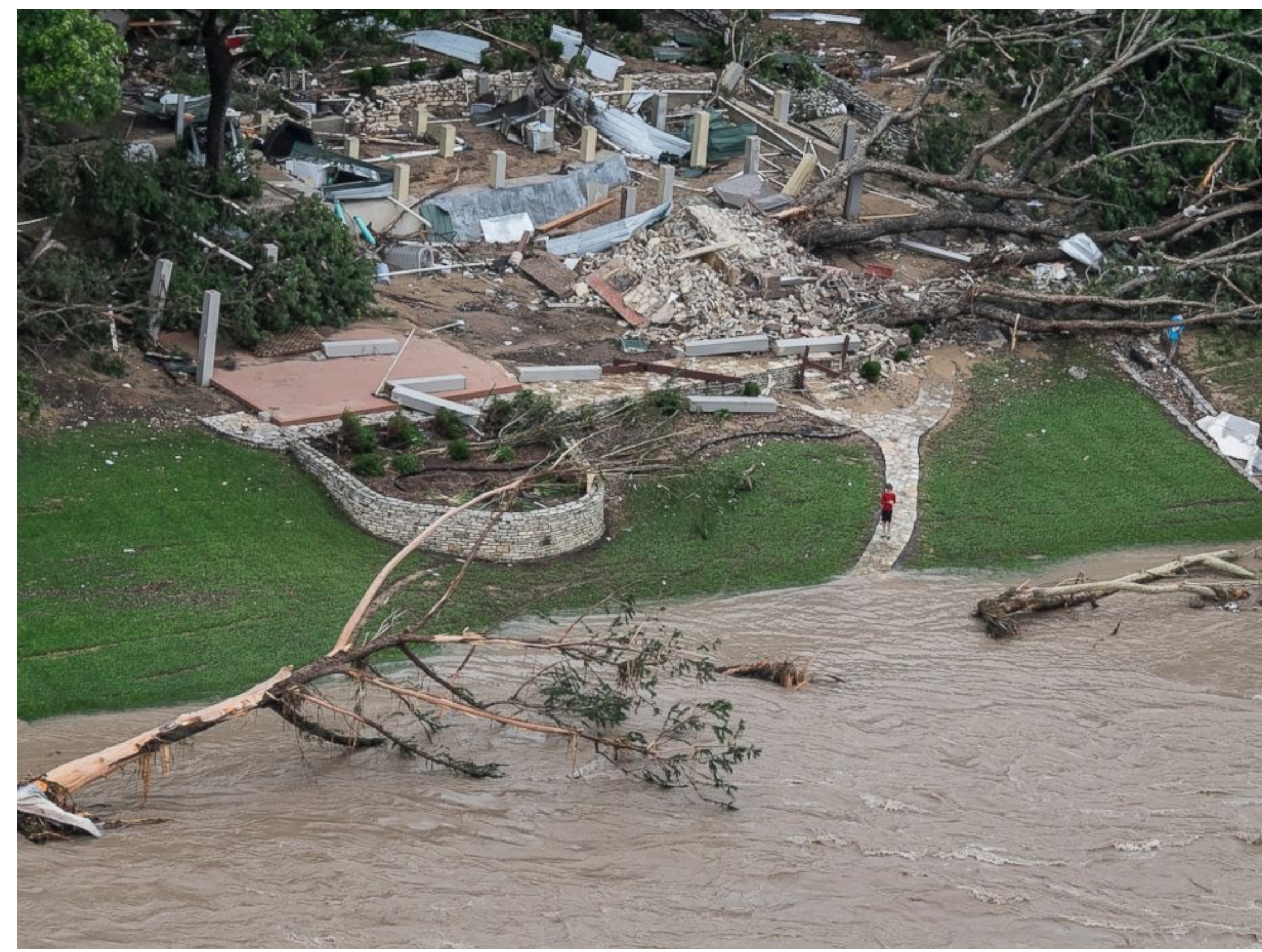
The Blanco River, TX, rose by almost 8 m in a day on May 24, 2015 during a flash flood, sweeping away roads, trees, and houses.
