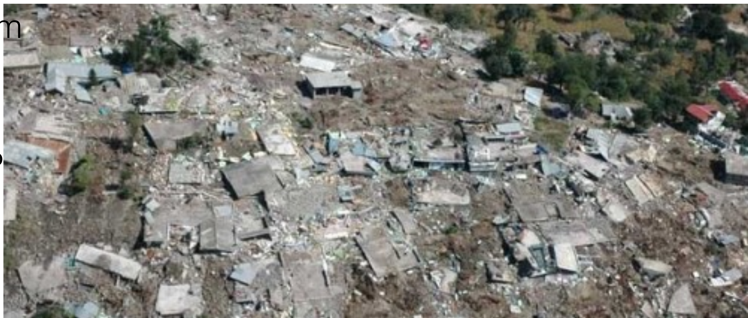
Destruction in Punjab, Pakistan Kashmir, caused by 23 seconds of ground shaking during the October 2005, M_w7.6 earthquake.
